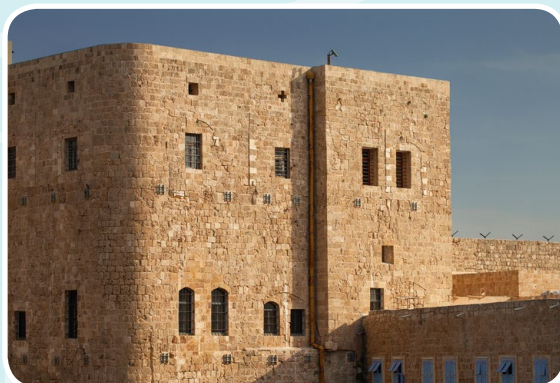
In 'Akká, Bahá'u'lláh was confined to this prison for over two years.
