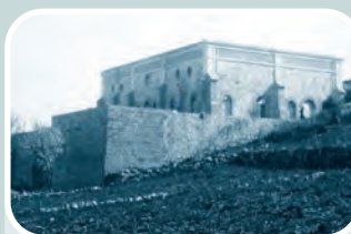
The Shrine of the Báb surrounds this simple structure.
